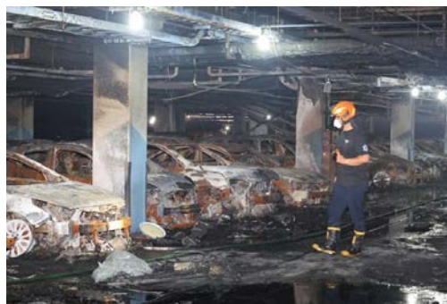
Figure 2. EV-caused fire in the parking garage in Incheon, Korea (The Korea Times, 2024)
