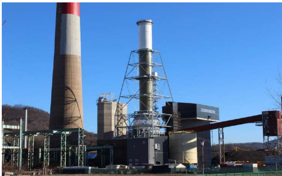
Figure 2. FGD plant of TPP Ugljevik
