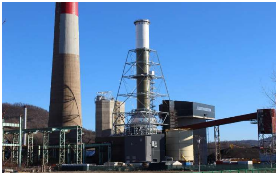
Figure 2. FGD plant of TPP Ugljevik
